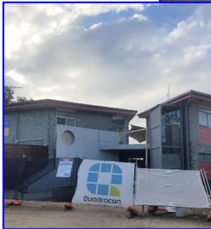
Photos of the clubhouse rebuild courtesy of Guy Bancroft
